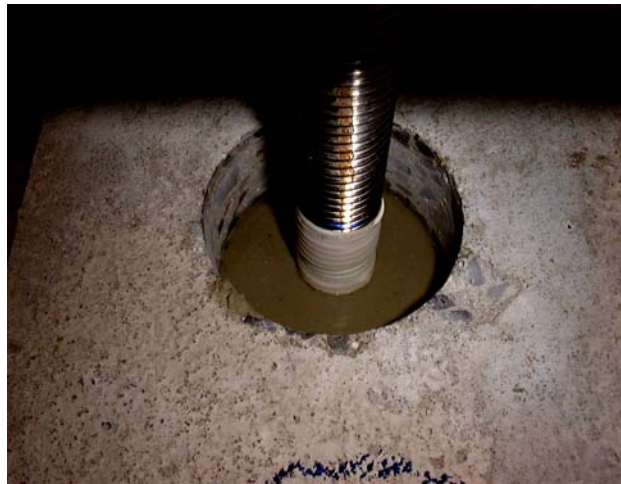
Picture 2: The upper anchorage area must be deducted mathematically from the anchorage length.
