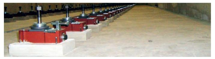
Positioned and grouted BW-Fixators®. Ready for machine arrival!
