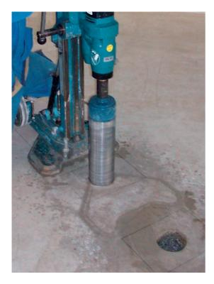
After marking the anchor holes, they will be drilled with a core drilling machine.
